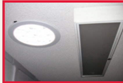
◀ New Solatube skylight at left, next to existing (off) fluorescent fixture
