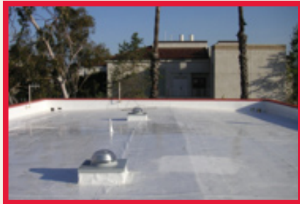
View of new Arroyo roof facing Aliso Hall
